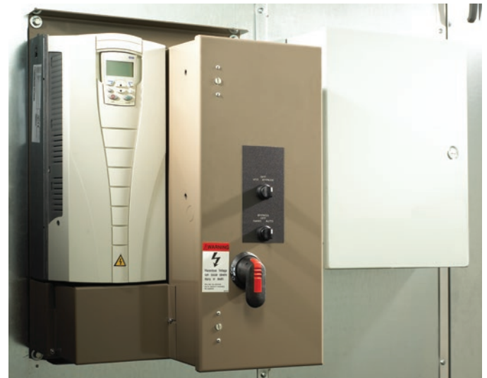
Variable-speed drives offer dramatic fan-energy savings.
