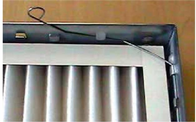
**FIGURE 108** - FULLY INSTALLED FILTER
