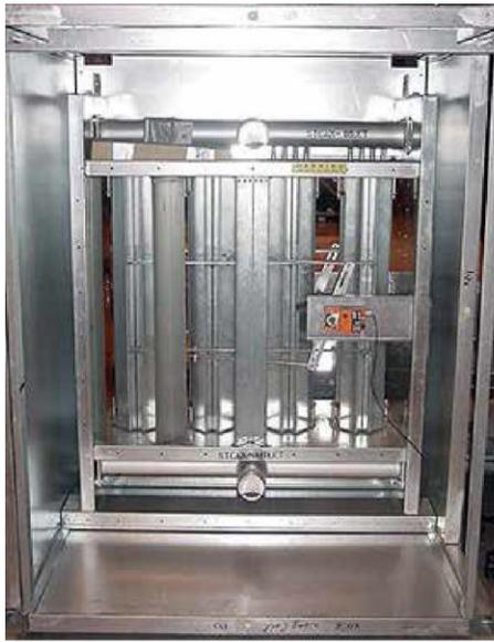
**FIGURE 84 - VIFB COIL (FACE-MOUNTED ACTUATOR SHOWN)**
