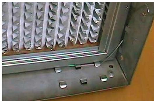
**FIGURE 111** - CORRECTLY INSTALLED CARTRIDGE FILTER
