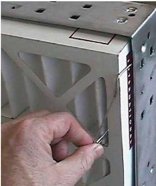
**FIGURE 110** - PLACE THE END OF THE LATCH OVER THE FILTER FRAME
