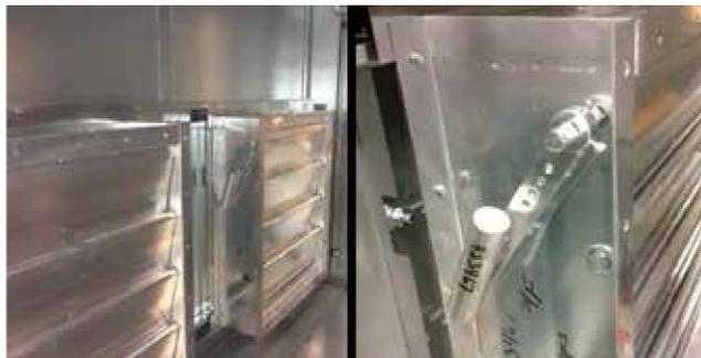
**FIGURE 50 - COUNTERBALANCE LOCKED INTO PLACE FOR SHIPPING**
