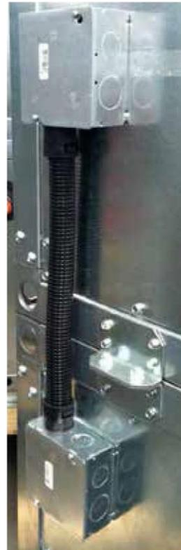
**FIGURE 29 - CONDUIT (P/N 025-39024-001) AND SJO CORD (P/N 025-35746-001)**
