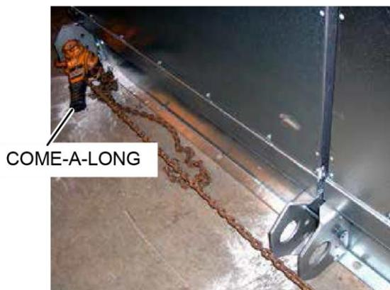
**FIGURE 33 - COME-A-LONG ATTACHED TO A SECTION**
