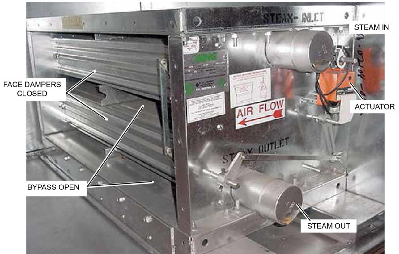
**FIGURE 83** - IFB COIL (HORIZONTAL TUBES AVAILABLE WITH STEAM AND HOT WATER)
