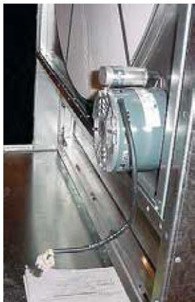
**FIGURE 65 - TYPICAL POWER WIRING OF ENERGY RECOVERY WHEEL**
