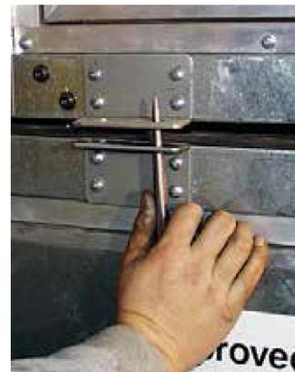
**FIGURE 44 - GUIDE BRACKETS TOGETHER**
