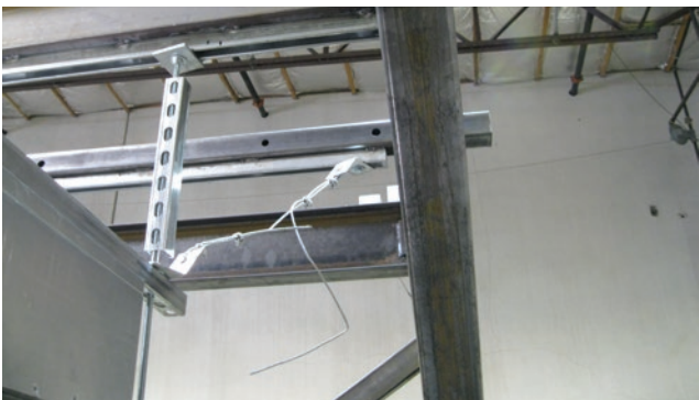
FIGURE 3 – LATERAL SUPPORT COMPONENTS FOR AHI 8-20
