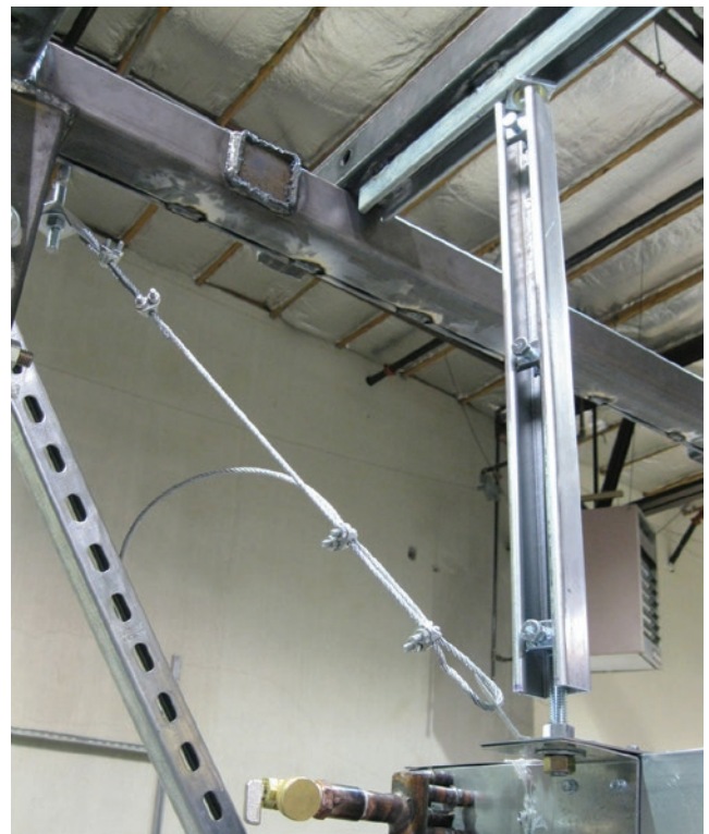
FIGURE 6 – UNISTRUT USED TO STRENGTHEN THE ROD.
