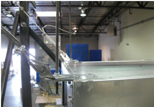
FIGURE 5 – OVERLAPPED FLAT, 90° AND 45° BRACKETS.
