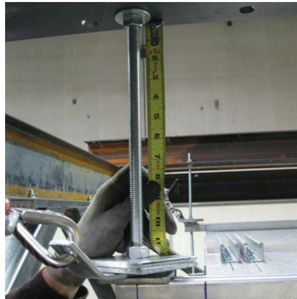
FIGURE 4 – RECOMMENDED LENGTH OF THREADED ROD
